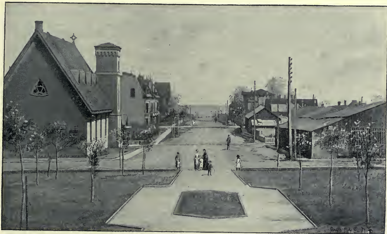
VIEW OF LEWING STREET, LOOKING NORTH.
